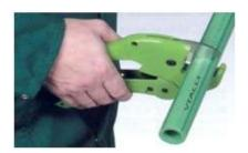
1.) Cut the pipe perpendicular to its axis
